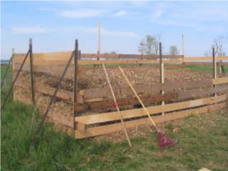
Figure 3. 2005 Composting facility on High Bluff Island.
